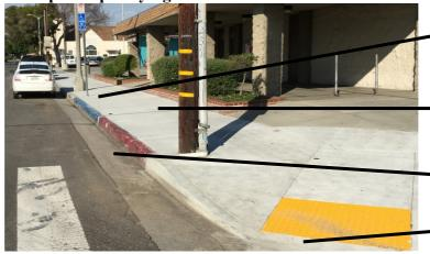
Doors can open and lifts can deploy because there are no obstructions adjacent to parking space.
